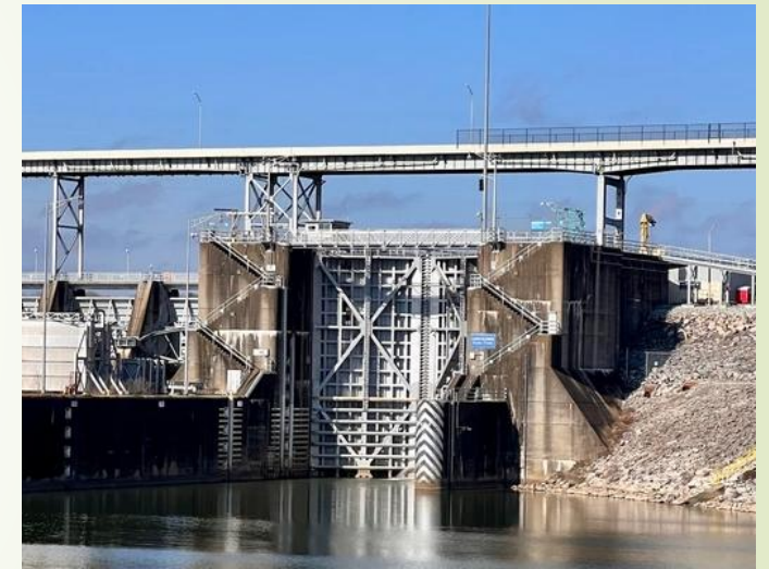
Watts Bar Lock
